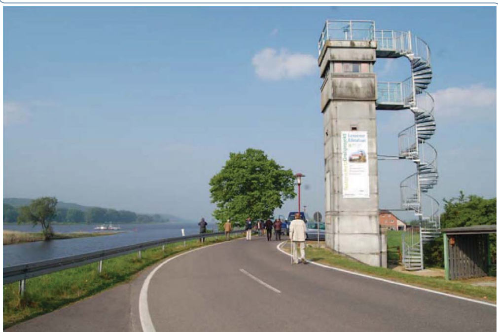
Figure 3.1. Former Border Police Watch Tower
